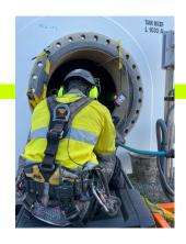
Conduct Rope access, CSE & Height safety operations for cleaning a 70,000,000L Petroleum Tank with a Vertidrive robotic UHP.
